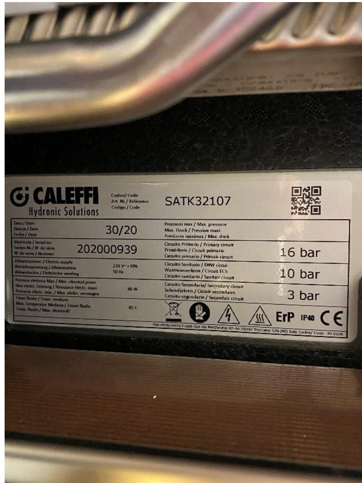
Figure 2-3 – Appliance Data Label
