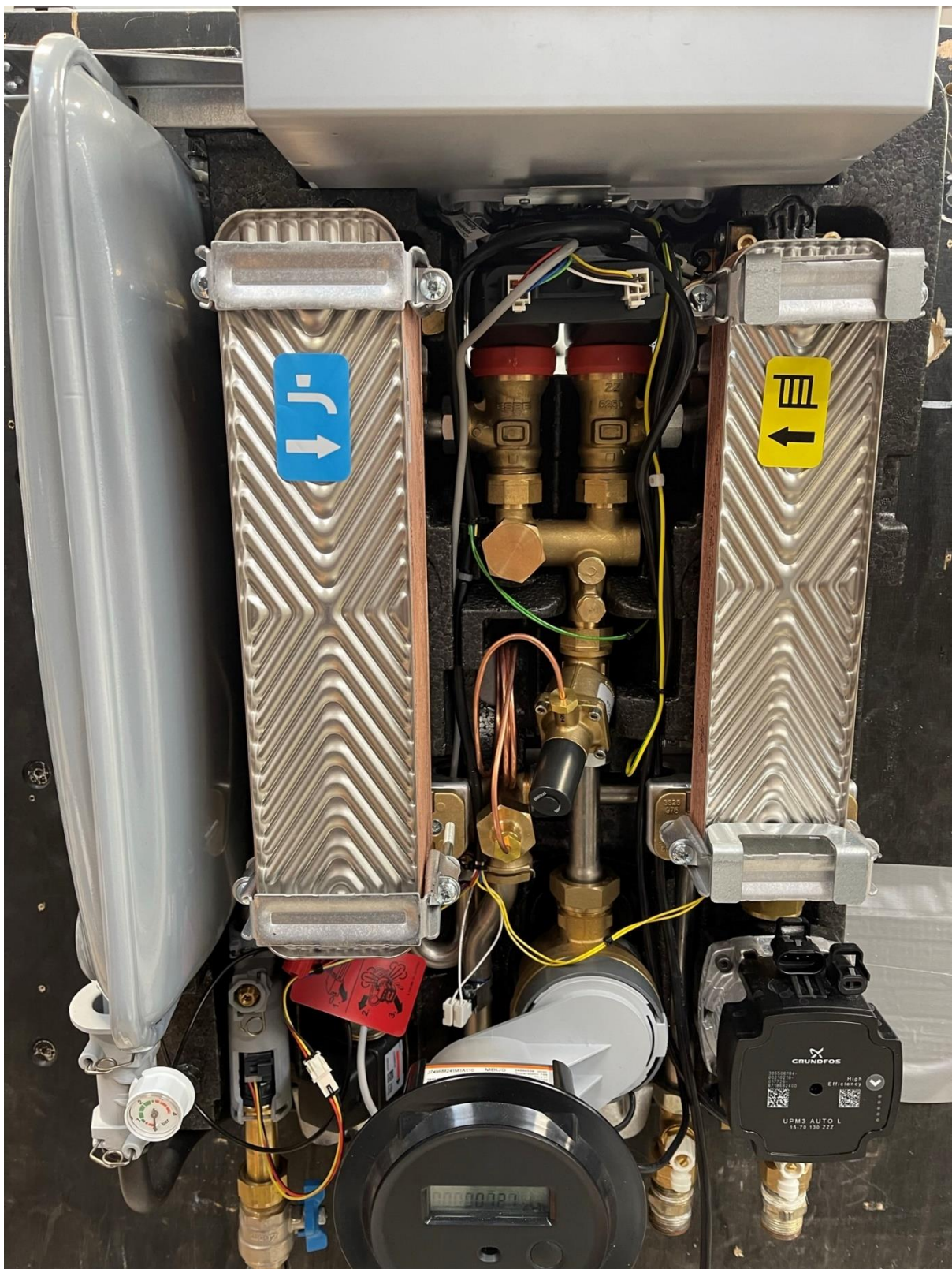
Figure 8.2 – Photograph of Appliance [Case Removed]
