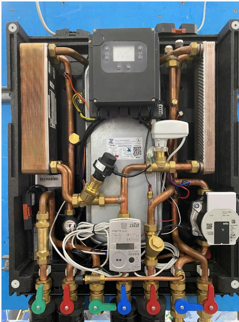
Figure 1 TI45 UL (Ultra Lean Electronic HIU), installed in the test rig
